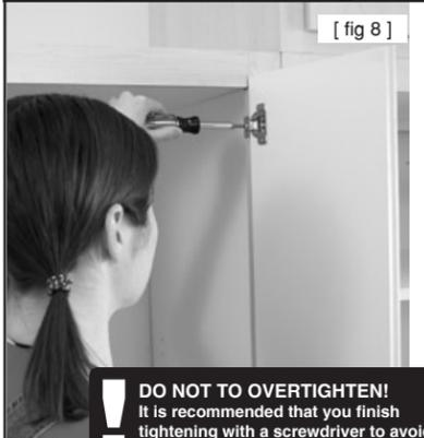
To hang doors, use the 1 1/2" silver screws. Hold door up so the door hinge hole lines up with the pre-drilled hole in the face frame. Screw in the hinge so the doors are level across the top and flush in the front. Take clear bumpers and attach as in fig. 8B, to top and bottom of doors.
